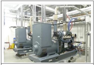
Two 350 kW Detroit Diesel engine gensets (above) were removed from the old powerhouse, remanufactured and "marinized" (cooling system modified for water heating).
